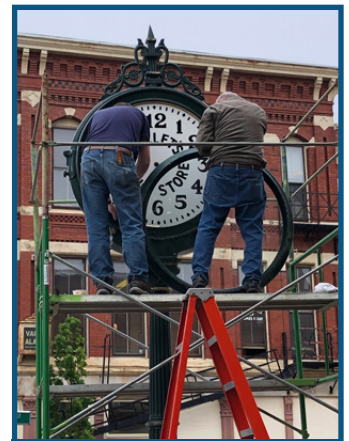
Making repairs to Hallett's Clock*
