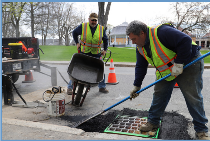
Hot top work on Washington Street
